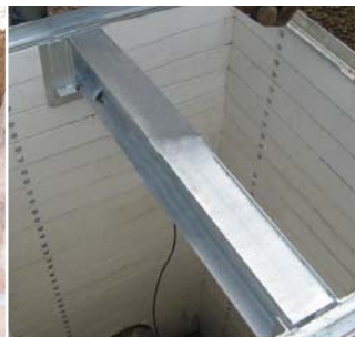
Deep water main
