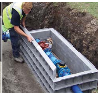
PRV installation
