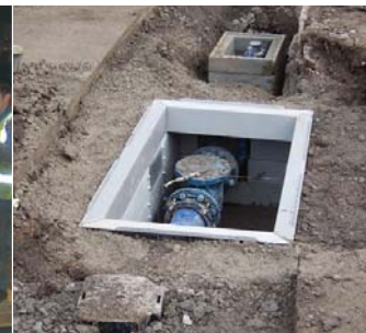
Corbelled water main
